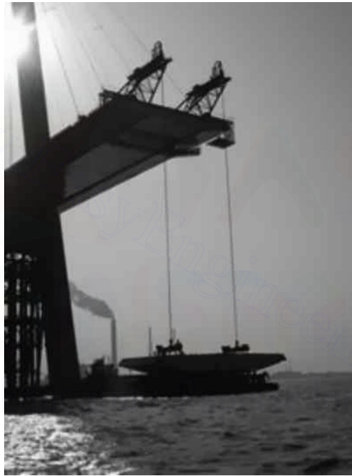
Figure 11.11 Lifting and erecting of one segment.
