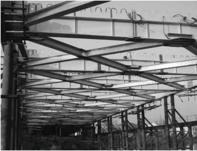
Figure 10.36 Rigid connections of Shang Xin Bridge.
