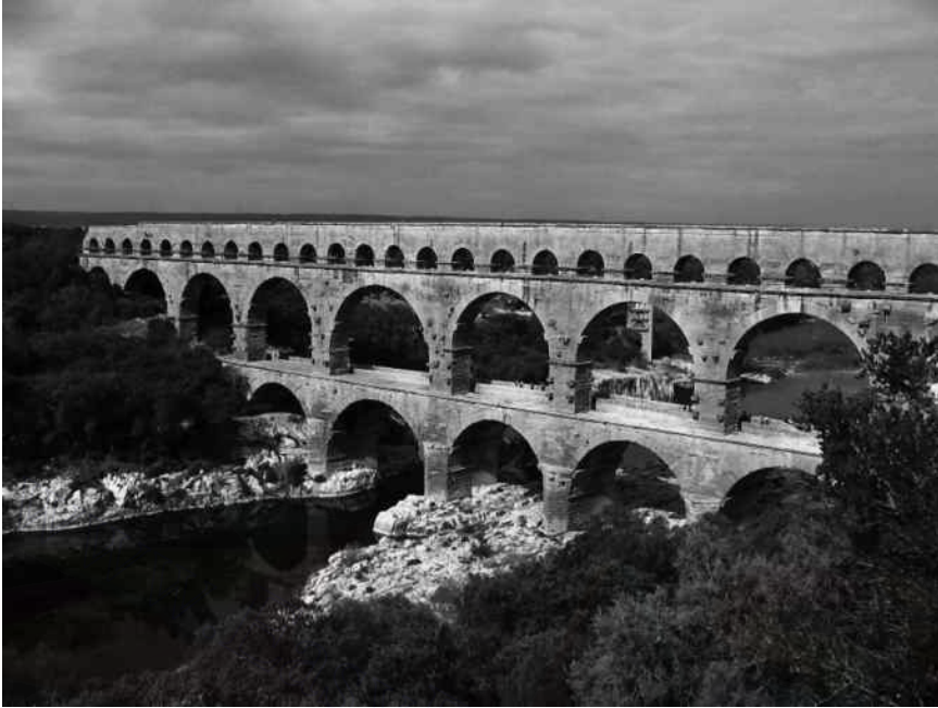
Figure 1.1 Roman viaduct, Pont du Gard, France. (Courtesy of http://en.wikipedia.org/wiki/File:Pont_du_Gard_BLS.jpg )
