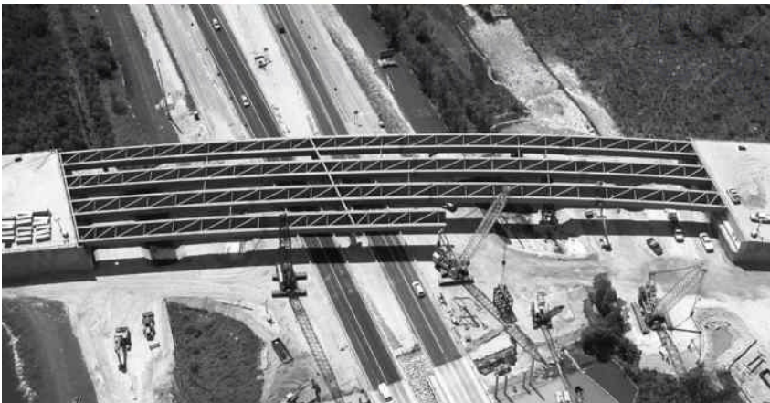
Figure 8.24 Top view of the Estero Parkway Bridge under construction.
