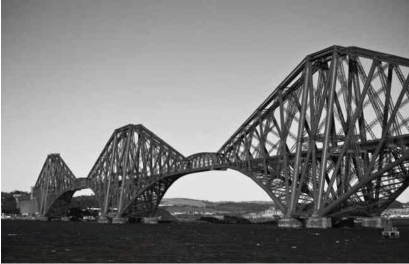
Figure 10.7 Forth Rail Bridge, Queensferry, Scotland.
