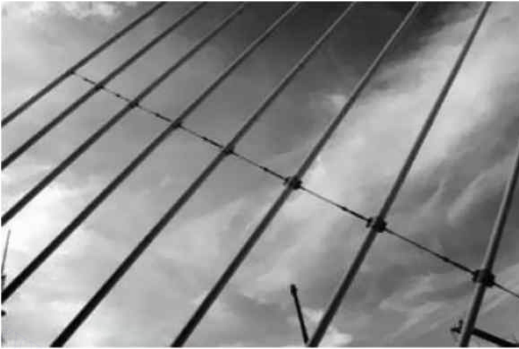
Figure 11.7 Crosstie of cables.
