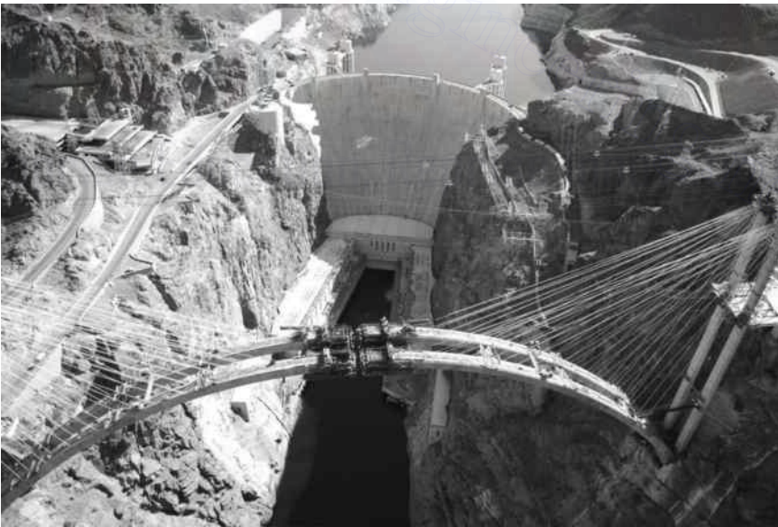
Figure 9.5 Cable-stayed segmental erecting of arch bridge. (Hoover Dam Bridge, Nevada, USA, Courtesy of galleryhip.com/hoover-dam-bridge-construction.html .)
