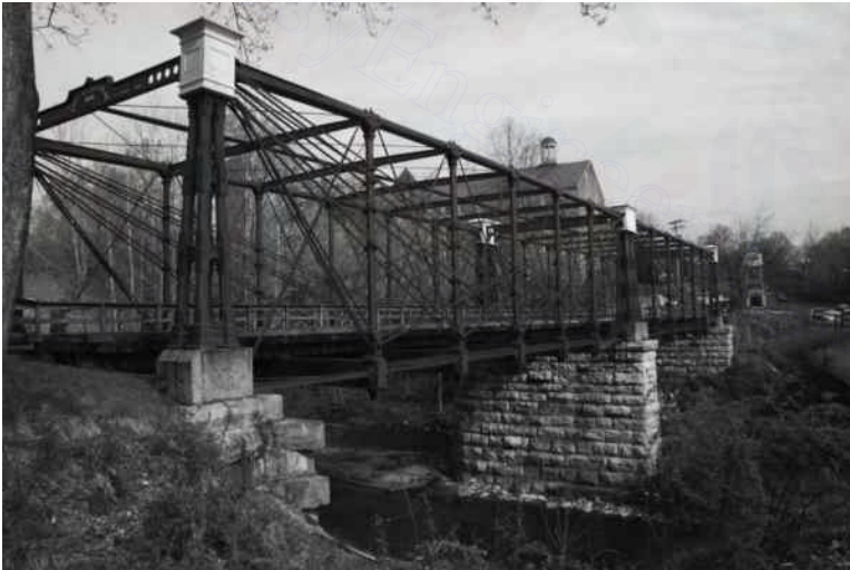
Figure 10.2 Bollman truss bridge.
