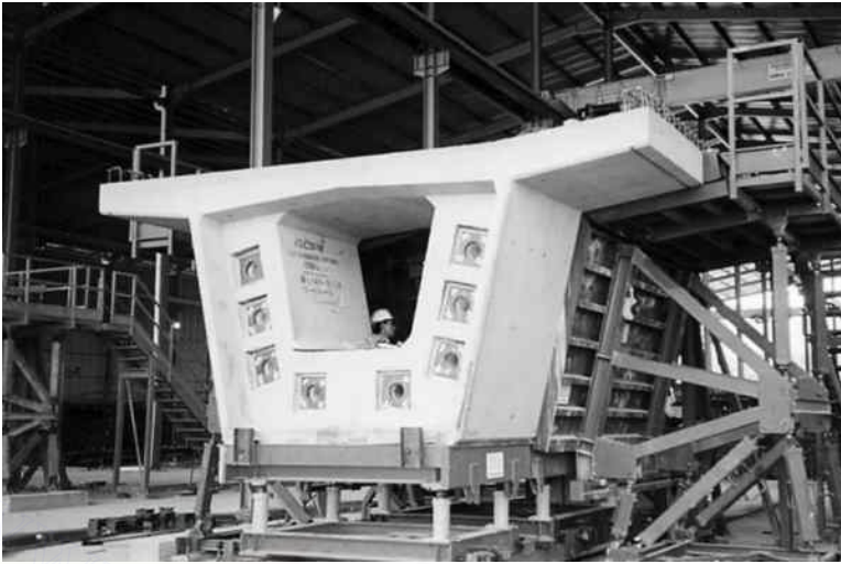
Figure 18.18 Adjustment of match segment and formworks for casting segment. (Courtesy of Ninive™ CASSEFORME, http://www.ninive.it/bridge-formwork/segmental-box-girder-forms/ .)
