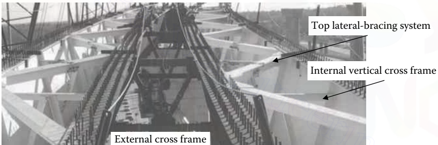
Figure 8.2 Twin-box girder bridge. (Courtesy of TXDOT.)
