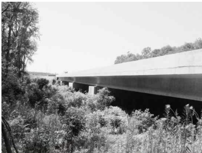
Figure 5.32 US23043 Bridge, Maryland.
