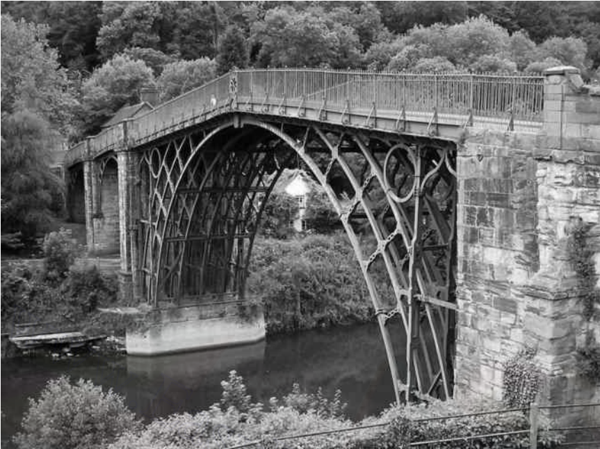
Figure 1.2 The first cast iron truss bridge at Coalbrookdale, Telford, England. (Courtesy of Tata Steel European Limited.)
