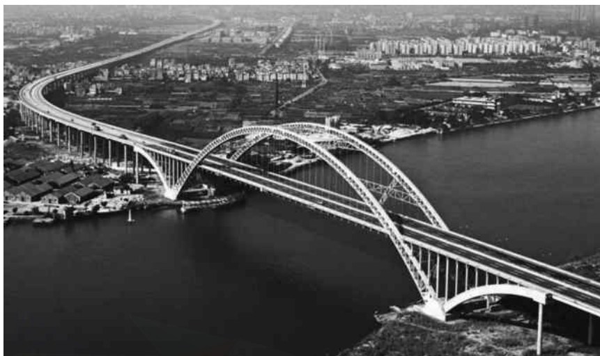
Figure 9.10 Yajisha Bridge, China, 2000, a half-through steel tubular concrete arch bridge with a main span of 360 m.
