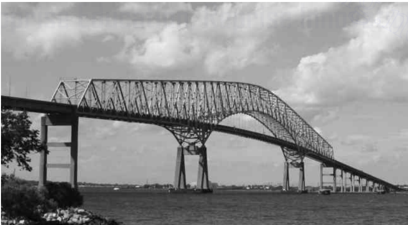
Figure 10.9 Francis Scott Key Bridge (I-695) in Baltimore, Maryland.
