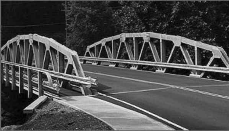
Figure 14.8 Pony truss bridge.
