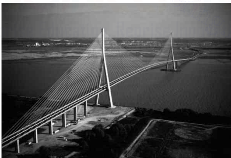
Figure 11.3 A cable-stayed bridge with auxiliary piers.
