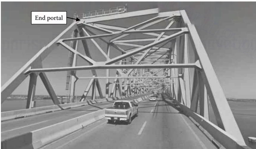
Figure 10.27 End portal of Francis Scott Key Bridge.
