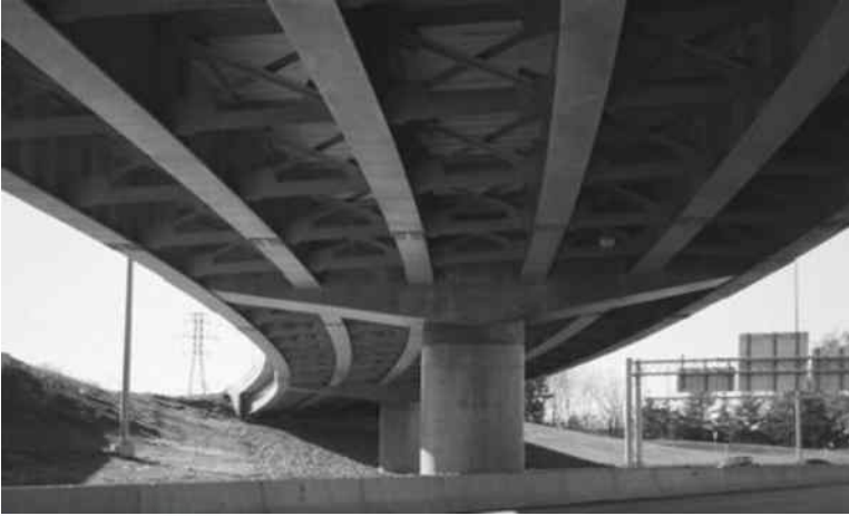
Figure 16.1 Integral pier on ramp FR-A over SR6060, Pittsburgh, Pennsylvania.
